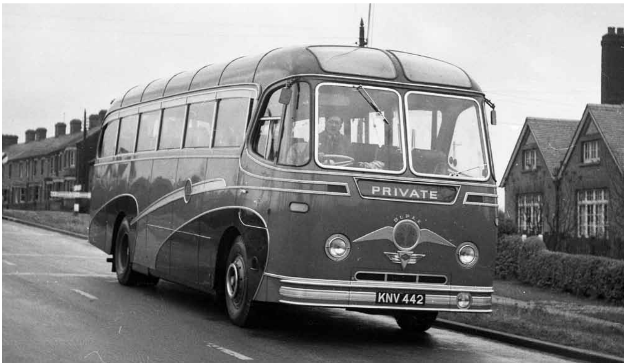
The Duple Elizabethan coachwork of KNV 442 looks quite substantial in this view of the A.E.C. Reliance coach taken at Daventry in 1957. (Photo courtesy R Marshall)
