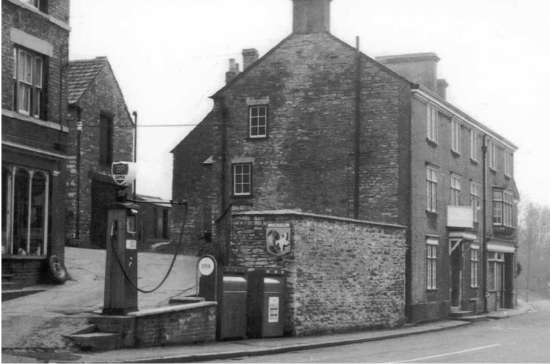
A view of the entrance to 35 High Street, Raunds showing its restricted access. The buildings to the right of the picture comprise the former Wheatsheaf PH and a number of cottages, the demolition of which both enhanced the site and provided road widening.
