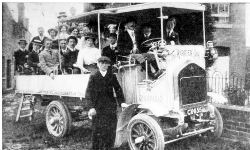
This photograph of CX 655 and that of CX 679 on the next page appeared in the trade press in February 1912. In this view CX 655 is in use as an excursion vehicle, fitted with cross-bench seating and a rear access ladder. (Photo courtesy Commercial Motor).
