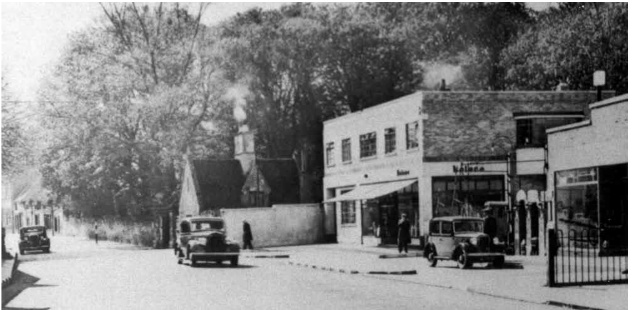
High Street South, Rushden in the early 1930s showing George Robinson's garage and showroom.
