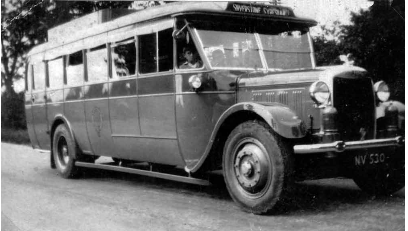
Another view of NV 530, Syd Kingston's substantial Gilford 168SD with Petty twenty-six seat coachwork, new in July 1931.
