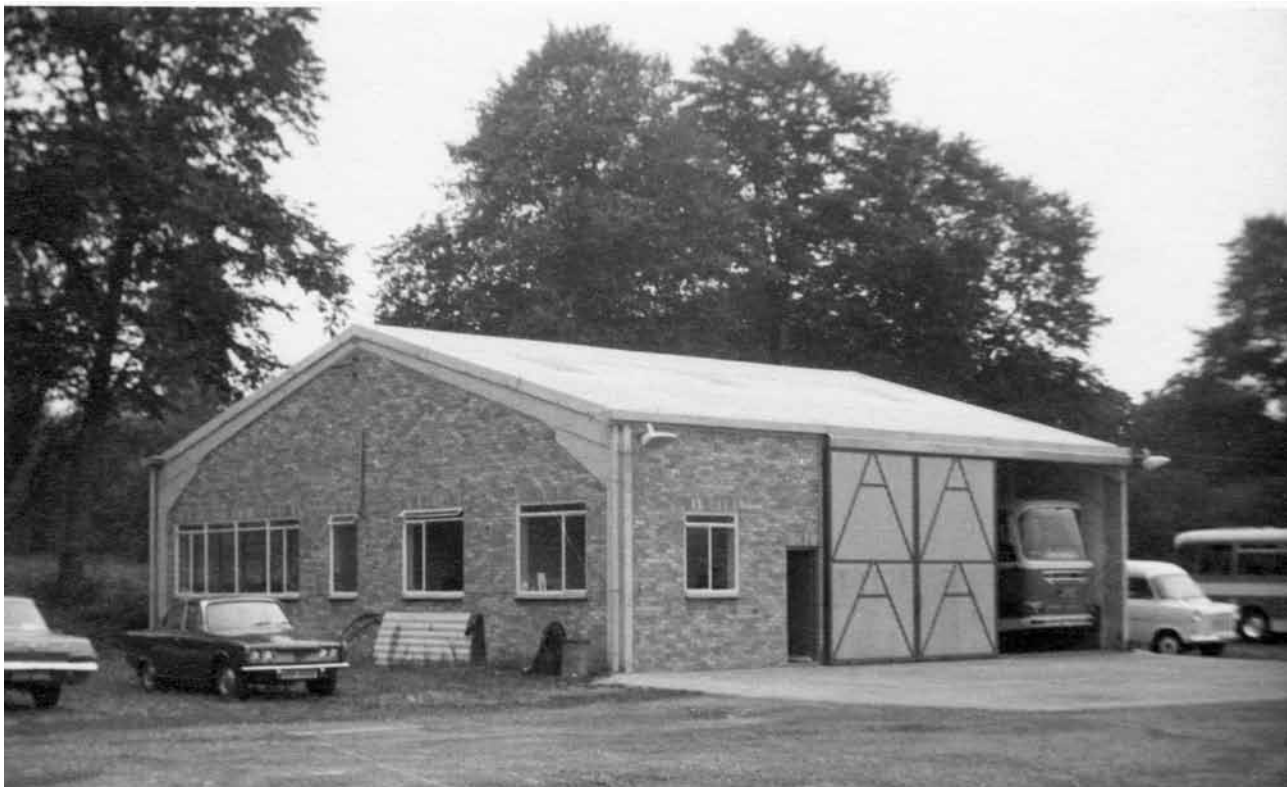
Jeffs' new Helmdon workshop building.
