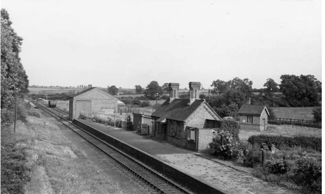
A view of Helmdon Station in 1951. The goods shed at the far end of the platform is still in situ. The main station building was accessed from the far side to provide partial cover for two coaches.
