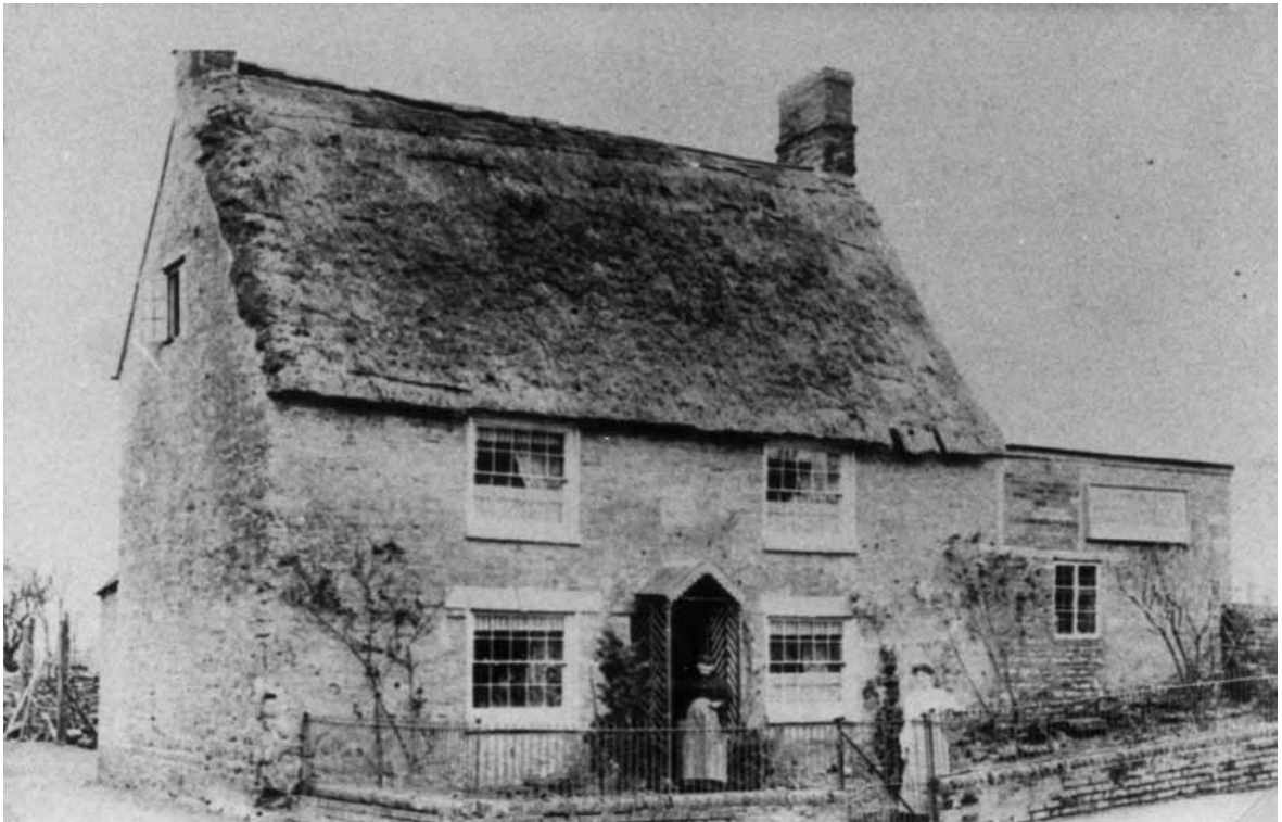
An early photograph of "The Rest" in Bradden Road, Greens Norton. The garage was built to the left of the property.
