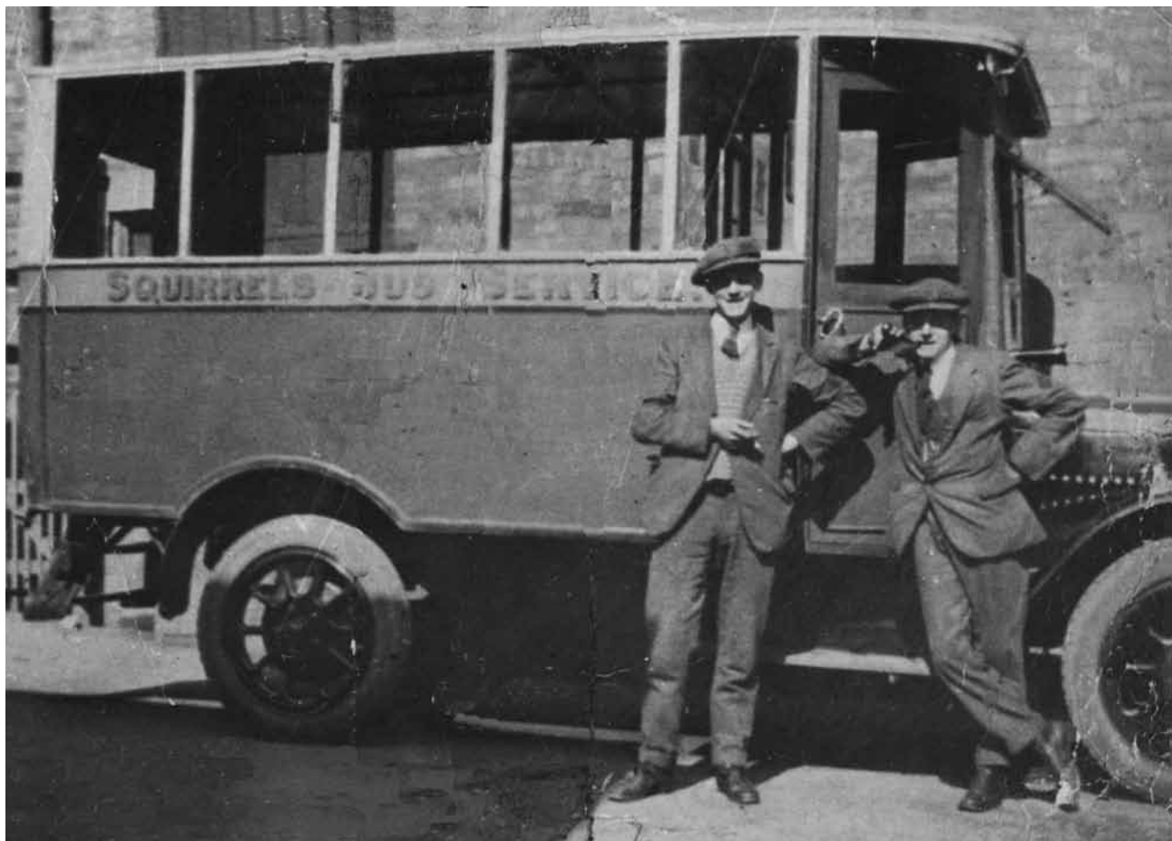
Benson's Morris single-deck which is said to have been fitted with a Billington body and on which the words "Squirrels Bus Service" can be seen below the windows.
