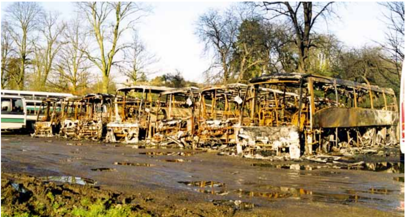
The scene of devastation at Helmdon depot following the January 2002 arson attack. From left to right are the remains of FE51 RHU; XWG 254; YFC 16V; P180 ANR; NBD 307V; NBD 304V and Y804 YBC. Leyland Leopard EWW 206T was also lost in the fire.
